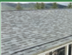
Intake Near Eave Edge
