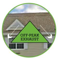
Multi Roll is a great solution for larger homes that have a large center beam or firewall, and cannot usually use ridge ventilation. Installing Multi Roll just off the peak, on both sides of the ridge, provides the right amount of exhaust.
