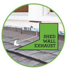
Many homes have roof-to-wall situations that are usually ignored. This can create hot spots in the attic. Multi Roll allows those areas to be vented properly, ensuring a cool attic and a balanced system.
