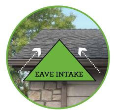
For a balanced system to work, every attic needs air intake; however, not every home is equipped with soffit vents. Multi Roll can be installed as an intake vent for homes with no overhang, too much overhang or tile roofs.
