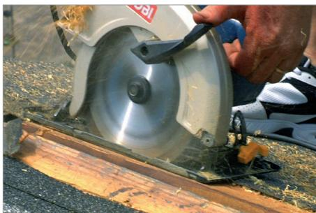
shingles covering the ridge are trimmed and removed, the ridge is ready for vent installation.
