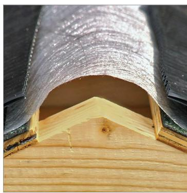
the corrugated plastic center section of the vent. Do this for the hip and ridge. This modified installation meets the requirements for UL790 "Class A"; standard installation meets the requirements for UL790 "Class C." Continue to Step 4.
