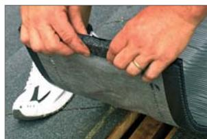
Vent along the entire length of slot also covering the 6" minimum uncut ridge on both ends. Bend vent into a "V" Shape. Secure at the lead edge after inserting
