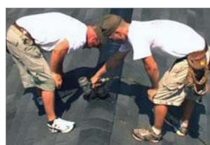
a coil nail gun can be used as long as the minimum penetration is  $\frac{3}{4}$ ". It is important when installing this vent that you maintain the pitch of the roof. The vent has been installed properly if the bottom of the vent is flat on the roof and the peak is slightly rounded.
