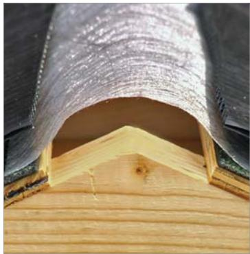
the corrugated plastic center section of the vent. Do this for the hip and ridge. This modified installation meets the requirements for UL790 "Class A"; standard installation meets the requirements for UL790 "Class C." Continue to Step 4.
